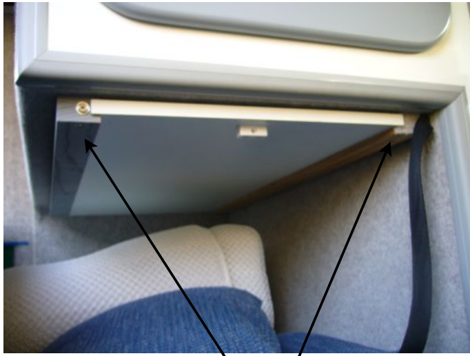
Hardwood runners routed to fit sliding top
